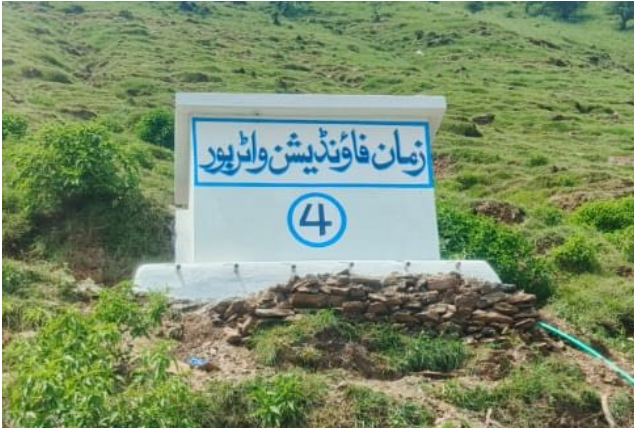
HAVELIAN: The water tank accompanying our fourth water bore project in Abbottabad.
